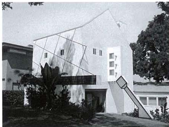
Figure 109. Eric Owen Moss, 708 House, Los Angeles, 1979–82. This house features supergraphics on its facade (now faded), a false gable (top right), and a protruding glass-paneled "flying door" supported by a steel "flying buttress" (lower right).
